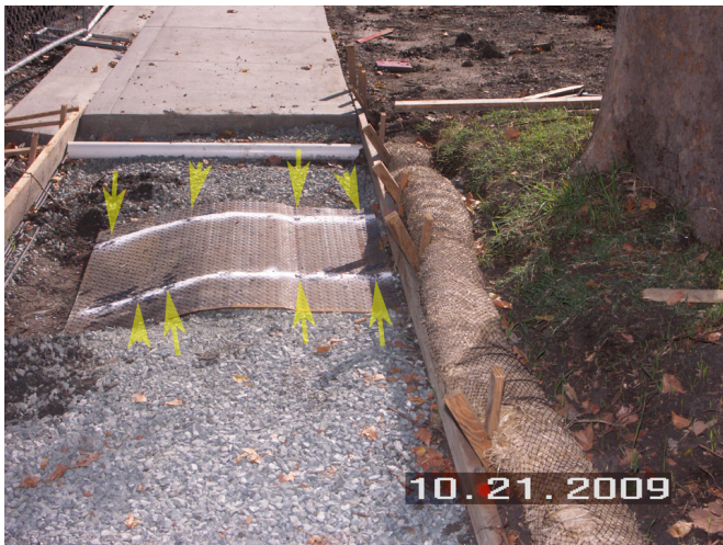
Image 15. Drill through the plate every foot or so, 1/4" to 3/8" holes for lag screws. The diameter of the lags, and length will be appropriate to the root diameter. Pre-drill holes in the roots for the lag screws. Fasten the plates tightly against the top of the roots with the lag screws. Then build the sidewalk.
