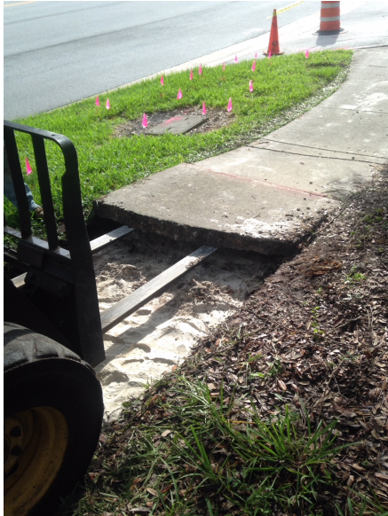
Image 5. Carefully remove sidewalk slabs that have been lifted by root growth.
