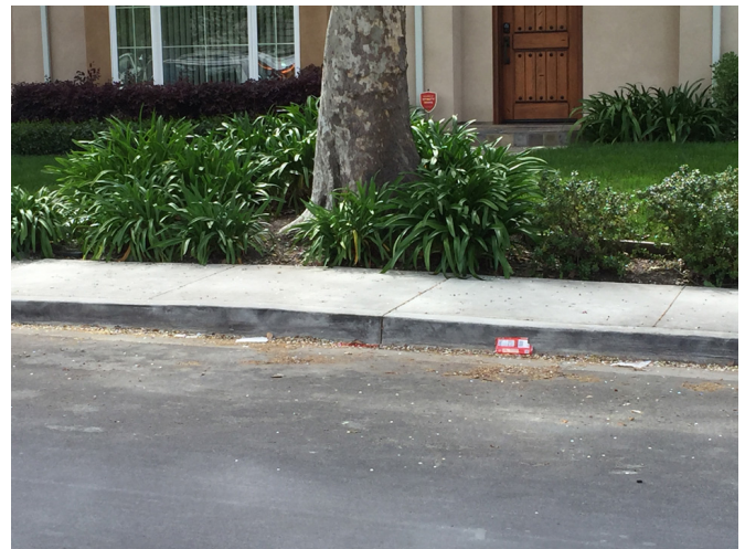
Image 16. Joe McNeil says, "Nine years later there is no disturbance lifting or fracturing of the sidewalk above the roots. The tree has looked great since, as well." The sidewalk and curb were elevated about an inch to accommodate the required thickness of the steel plates.
