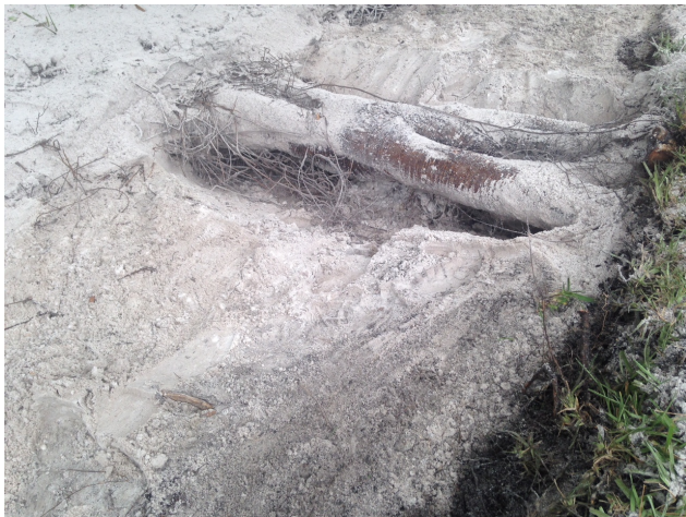
Image 7. Locate the major roots that are lifting the sidewalk.
